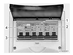
Fig. 101 Safety cutout and FI-switch (230 V fuse box)
