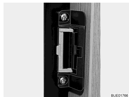
Fig. 152 Locking device (ventilation position)
