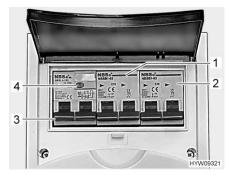
Fig. 102 Safety cutout and FI-switch (230 V fuse box)
