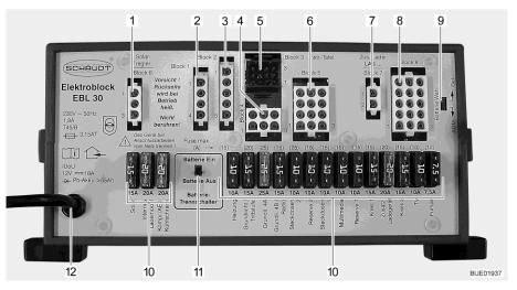
Fig. 95 Transformer/rectifier (EBL 30)
