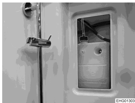
Afb. 164 Buffertank (warmwaterverwarming)
