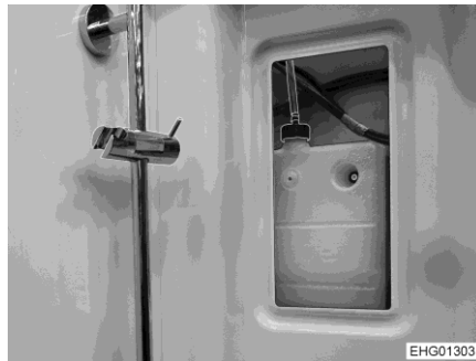
Afb. 222 Buffertank (warmwaterverwarming)
