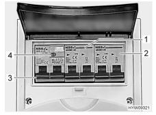
Fig. 155 Safety cutout and FI-switch (230 V fuse box)
