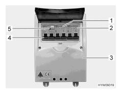
Fig. 146 Safety cut-out and FI-switch (230 V fuse box)
