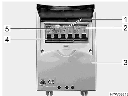
Fig. 70 Safety cut-out and FI-switch (230 V fuse box)
