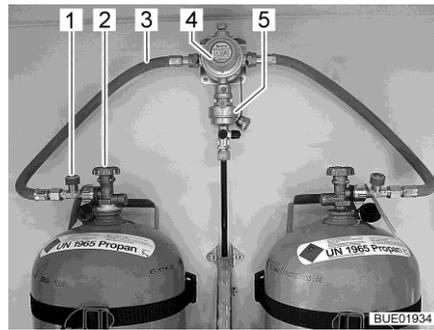
Fig. 83 Gas bottles with DuoControl
