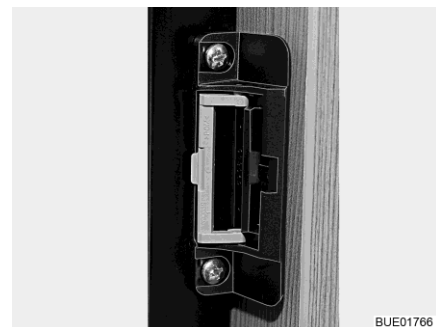
Fig. 152 Locking device (ventilation position)
