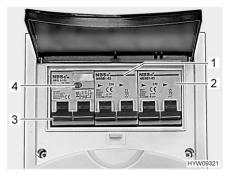
Fig. 111 Safety cutout and FI-switch (230 V fuse box)
